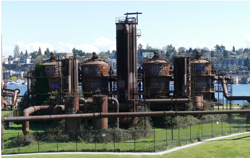
Vintage gas works now public art installation in Seattle, Washington.
